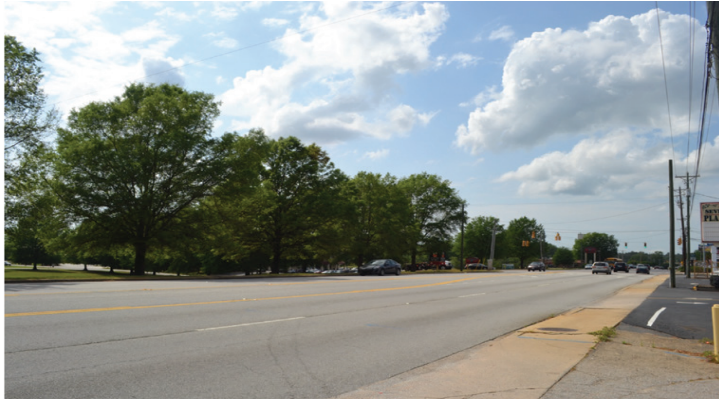
Sidewalk along St. Andrews Road approaching the intersection at Piney Grove Road.
